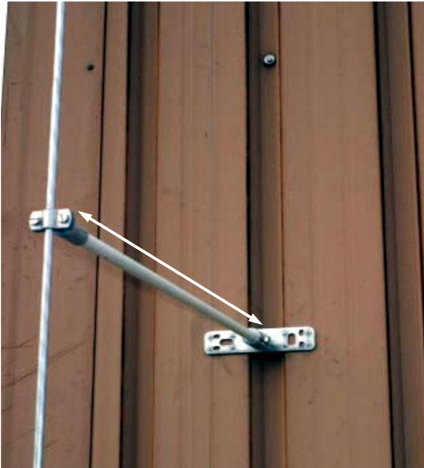
Installation of the distance holder
