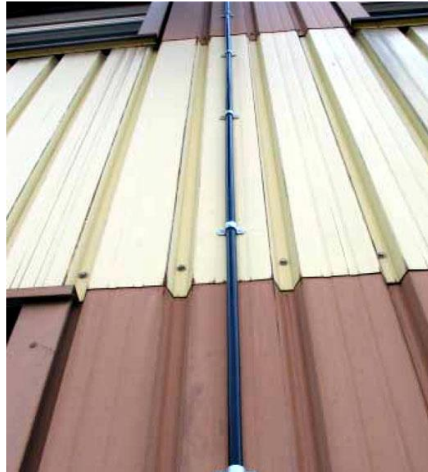
HVI ® conductor installation
